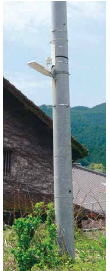
▲整備が進む防犯灯
